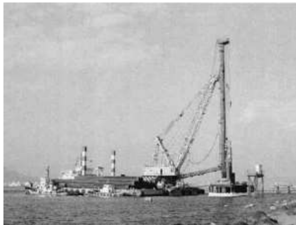
Photo 3 A view of construction
